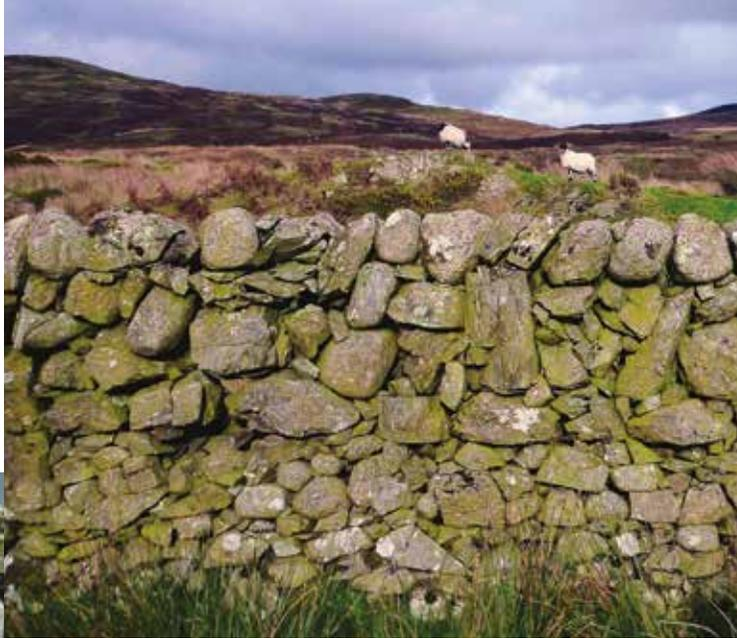
**GALLOWAY DYKE** (above) Also known as a 'half and half' dyke. This style of dyke is built with a double dyke at the bottom and a single dyke above. Common in sheep farming areas, the solid base provides shelter from the weather for the animals, while the 'tottering' appearance of the top half reduces the temptation of sheep to jump on or over it.
