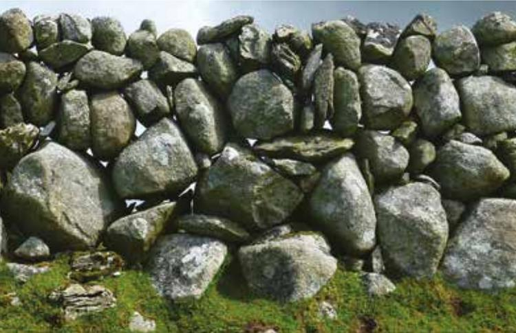
**SINGLE DYKE** (above) Where large irregular stones are abundant, the dyke is built such that single stones create both faces of the wall. Where large rounded stones are used, it is usually then called a Boulder Dyke. This style of building often has noticeable gaps between the stones and is most common in upland areas.
